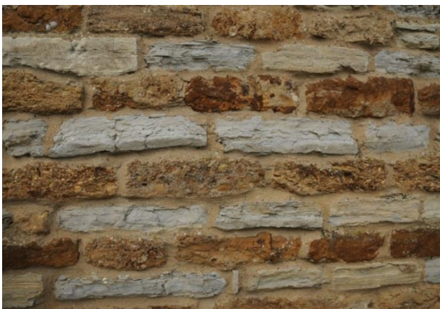
Left: A stone wall with alternating courses of Ironstone and Blue Lias and recent grey flush/brushed sharp sand/cement mortar.
