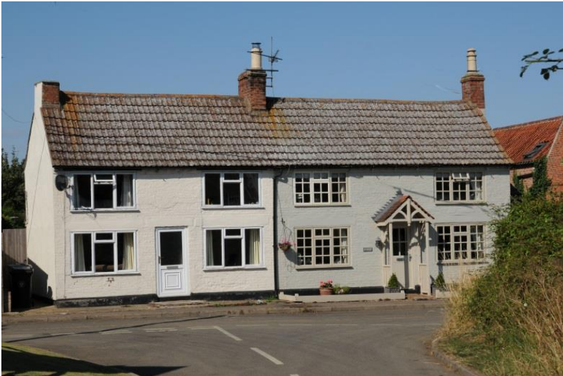
4: Pair of C18/19 cottages, rendered. 3 chimneys, pantiles replaced with concrete interlocking tiles. Original openings enlarged and atypical windows installed.
