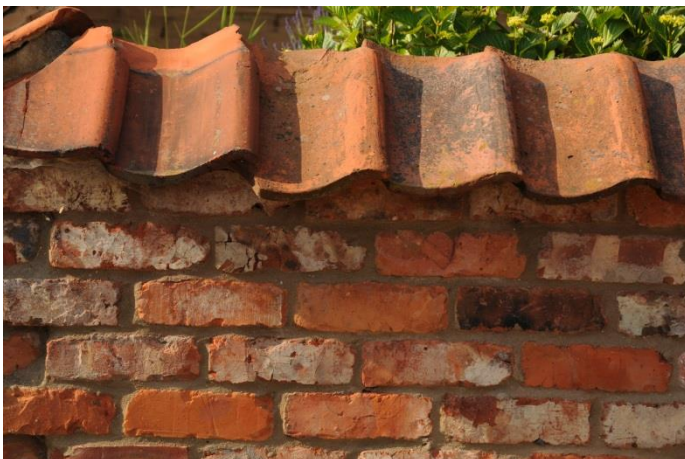
Left: Recent garden wall using reclaimed red and white (painted) bricks. No coursing, using metal ties under reclaimed clay pantile coping . Little vernacular justification for this.
