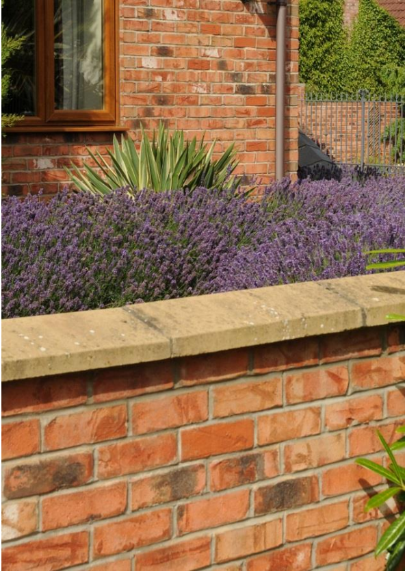
Left: Recent garden wall using traditional mixed red brick (metal ties - no bonding) and pale mortar under concrete “stone” coping stones. Flush pointing.
