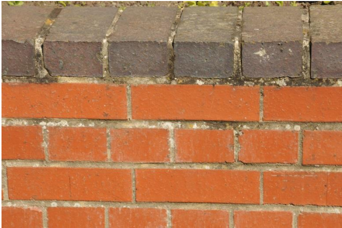
Left: Modern (flood protection?) wall built from red engineering class bricks, in English Garden Wall bond , with alternating header/stretcher courses under blue brick coping
