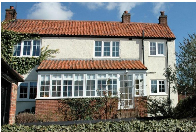
3: Possibly C18/19 formerly a Blacksmiths. Rendered but pantile & chimney. UVPC windows. Front extension, with pantiles but otherwise glazing is dominant.
