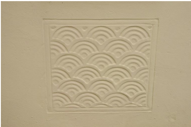
Left: Rendered and painted house wall with pargetted panel for interest (rather than function). Attractive, but out of context with vernacular.
