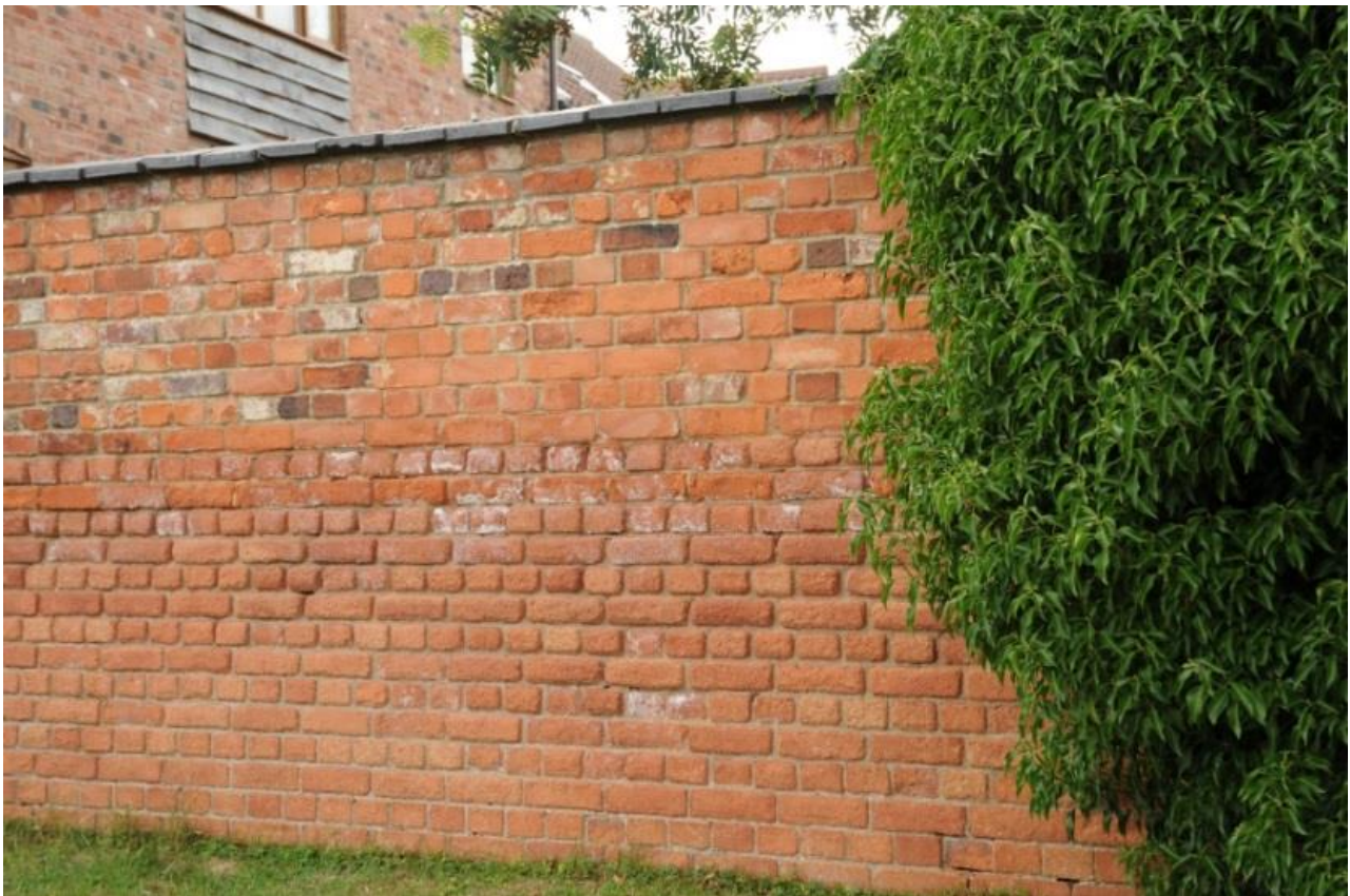
Above: C19/20 garden wall, (heightened) red brick English Garden Wall bond; lower alternating header & stretcher courses, upper uses headers on 6 th course. Blue clay coping stones
