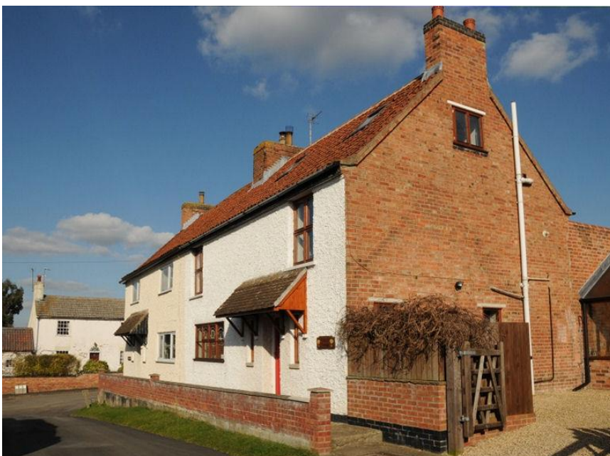
3: Two prominent cottages. Typical pantiles, chimneys & brick gable. Front elevation rendered & porches added, but character remains. Concrete coping on front wall is atypical.
