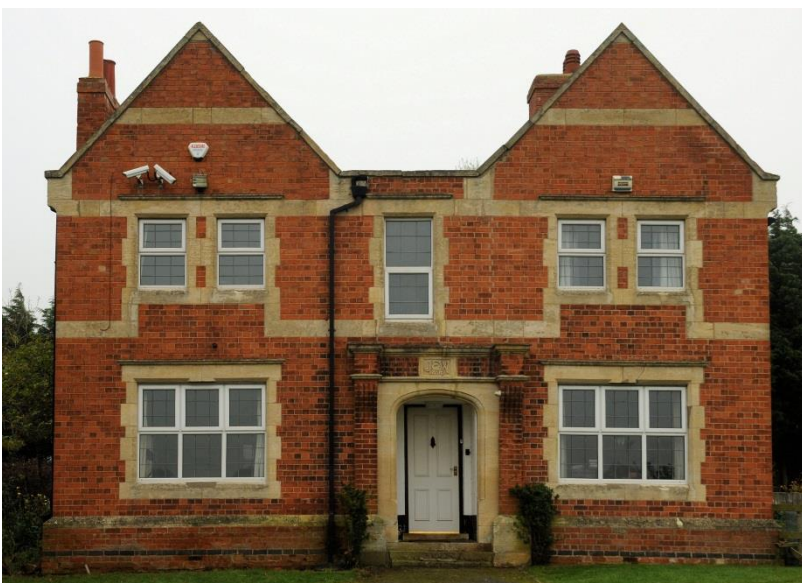
1: Date stone 1890. Larger C19 “Villa” Red brick with distinctive cream brick & stone banding and a portico. Gabled “M” shaped roof with eaves detail & tall chimneys, assumed slate roof. A one-off.
