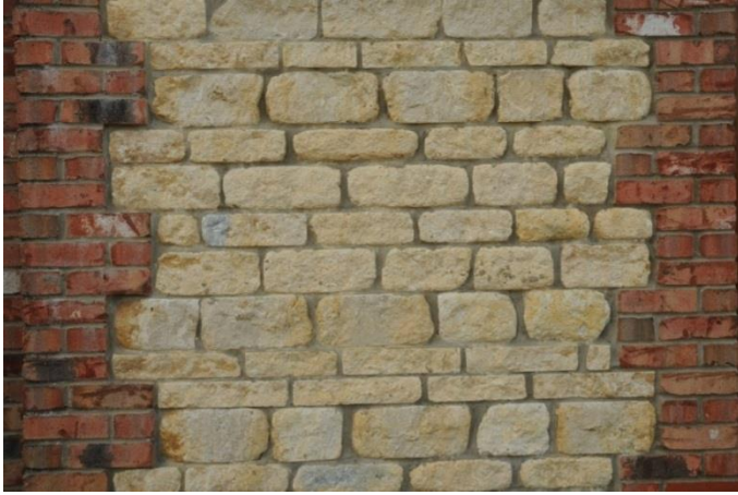
Left: Typical reclaimed brick wall but with recent limestone . Stone rough-dressed, laid with regular header courses. Reflects from façade on new buildings in Back and Tow Lane.
