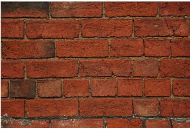
Left: Traditional red brick house or garden wall with coursing using English Bond with headers on every 5 th or 6 th course and recessed narrow, pale mortar/pointing.
