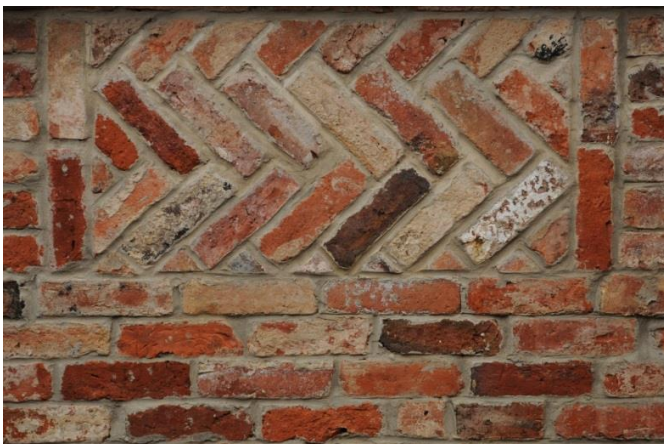
Left: Recent house wall using reclaimed brick with panel for interest (rather than function) using bricks on end and herringbone. Attractive, but out of context with vernacular.
