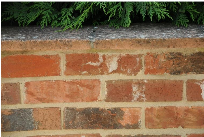
Left: Recent low wall using older mixed red brick with weathered concrete coping slabs and smooth pale mortar, flush pointed.
