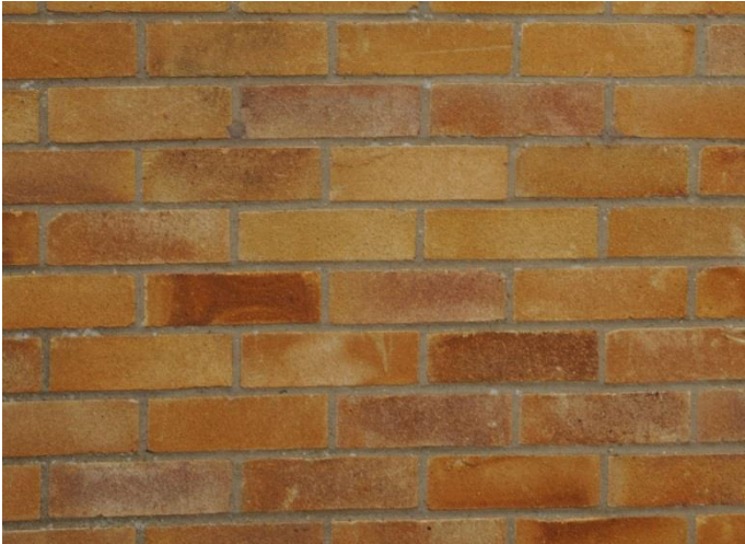
Left: Modern wall; bricks laid using metal ties and no headers. Predominantly buff/pale brown bricks and contrasting grey (mortar bucket handle pointed) is not typical of village.
