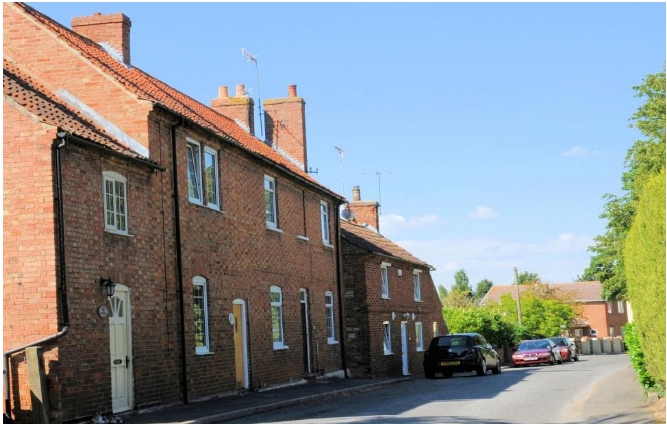
5: Paired cottages (next to 3; taller & setback). New extension. Red brick & regular pale headers. Pantiles & chimneys. New stained timber casement windows in original openings.
