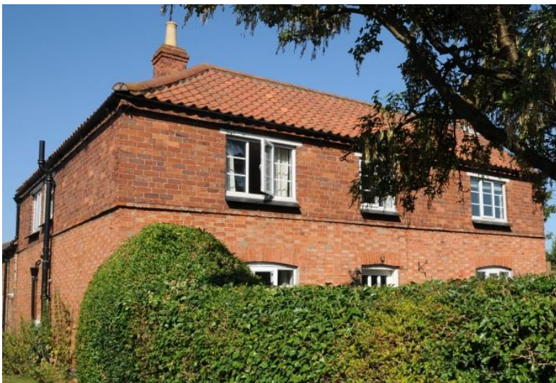
1: C18/19 farmhouse. Brick & pantile 3 chimneys (hip/gable). Lower walls red & pale “Chequerboard,” dentil course, upper walls larger mixed red bricks. Original openings with casements, blue tile sills and brick/stone lintels.
