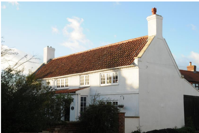
6: Cottage C18/19 formerly a bakery. Although gable end is sideways on to the road this is a prominent cottage may have been two originally. Although rendered the gable end is stone along with the rest of the house.
