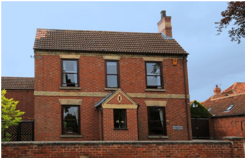
5: Prominent Farm house & outbuildings. Red brick & paler headers & cream bands. Newer porch. Brick wall with blue on-end coping. One chimney removed. Concrete tiles.
