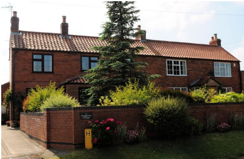
4: Pair C19 cottages (4 originally). Red brick, pantiles & 4 chimneys. Porches & front wall (red brick, with blue on-end coping) added. Replacement casement windows, atypical.
