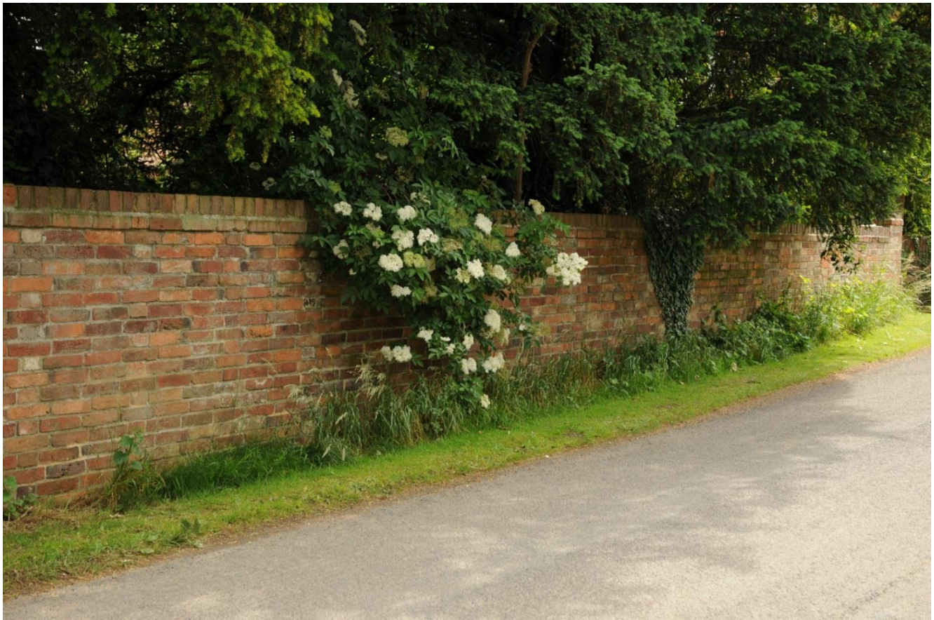
Above: Traditional (C19/20) garden wall with mixed red bricks laid in Flemish bond with 5 stretchers to one header. Brick on edge coping on top of wider final course of stretchers
